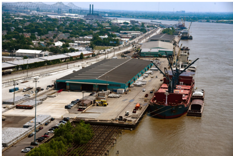
Louisiana Avenue Terminal
